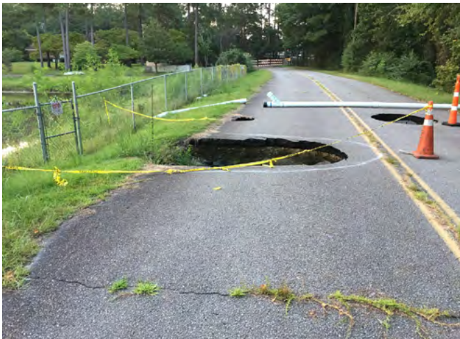
Figure 5 Springwood Lake Dam – September 4, 2018
