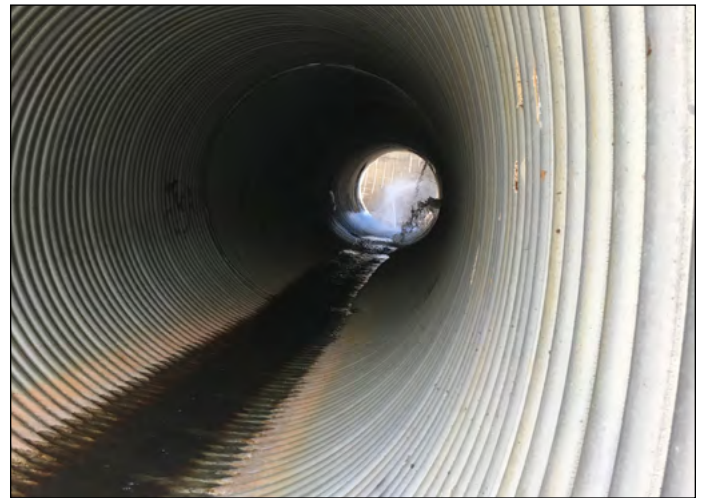
Figure 3 Upstream View of Springwood Lake Dam Auxiliary Spillway Discharge Conduit – March 21, 2018
